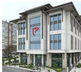
GÜNGÖREN MUNICIPALITY BUILDING Istanbul
