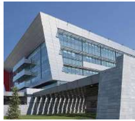
Istanbul Airport IGA DATA CENTER Istanbul
