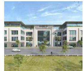
BAĞCILAR BELEDİYESİ BUILDING Istanbul
