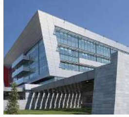
Istanbul Airport IGA DATA CENTER Istanbul
