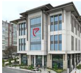
GÜNGÖREN MUNICIPALITY BUILDING Istanbul
