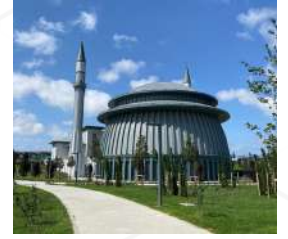
Istanbul Airport ISTANBUL AIRPORT MOSQUE Istanbul
